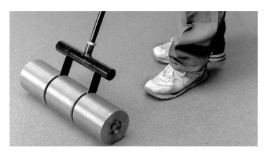
Roll slowly with a 100 lb. roller. Roll in both directions and avoid trapping air.
