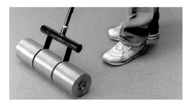
Roll slowly with a 100 lb. roller. Roll first from the center out so air does not get trapped under the material, then roll lengthwise.
